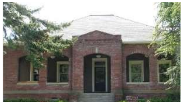
A conversion of a historic guardhouse in Fort Ward retains the historic façade and detailing of the original building.
