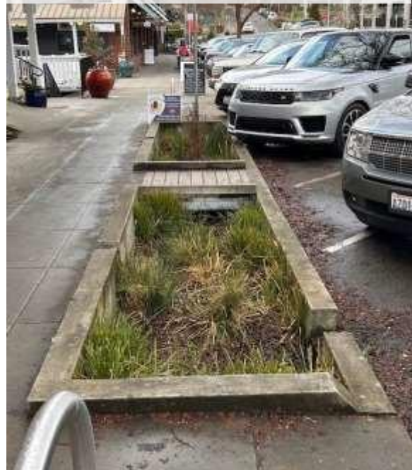
Winslow Way stormwater treatment ensures water quality and resilience to flooding within the public right of way.
