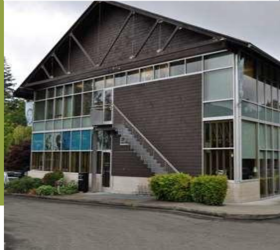
An office building on Hildebrand Lane in Bainbridge Island uses detailing and alternation of two primary materials to create a sense of texture and human scale.
