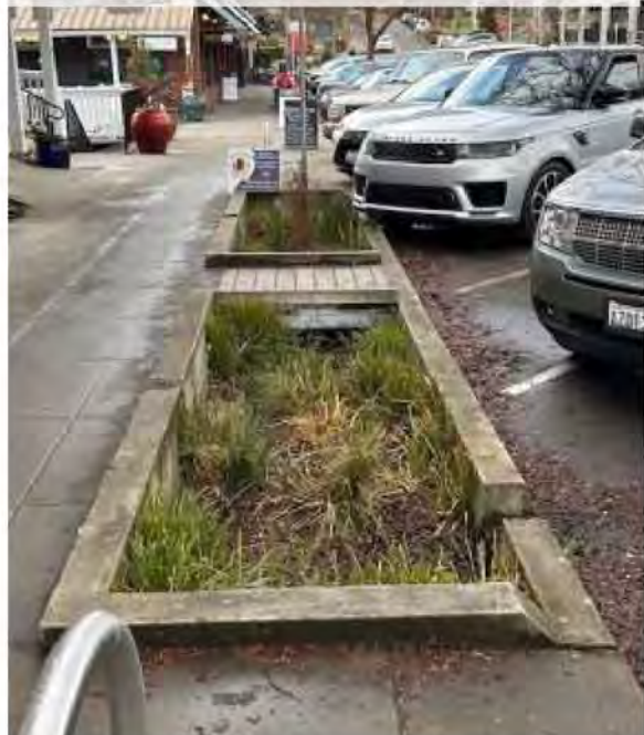
Winslow Way stormwater treatment ensures water quality and resilience to flooding within the public right of way.
