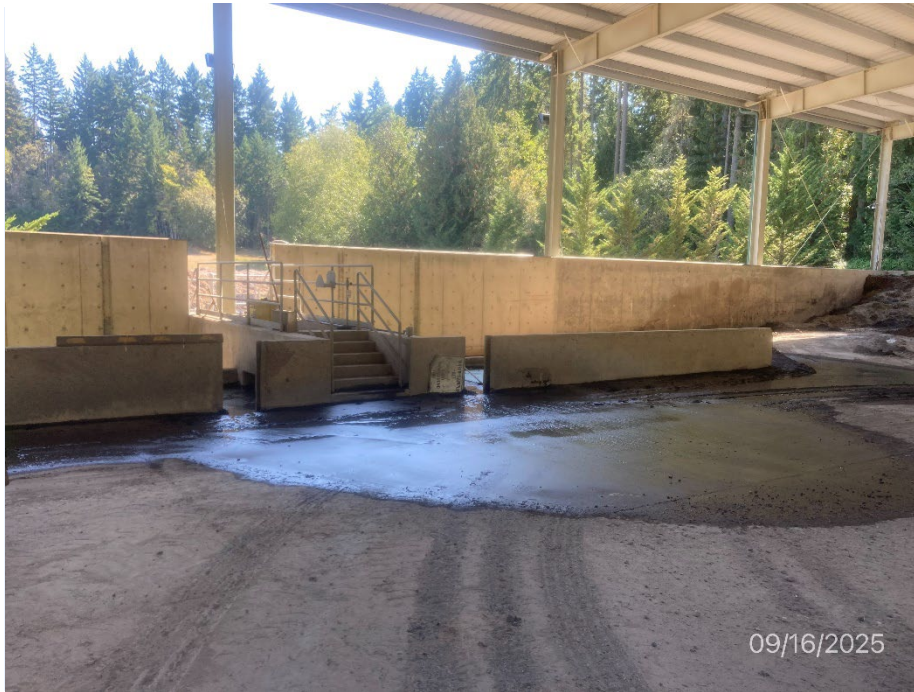
Photo [3] Description: Decant tipping floor.
